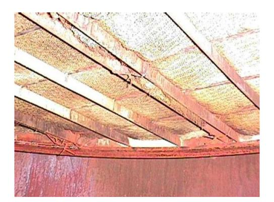
Here is an Ethylene plant caustic tower, with fouling.
