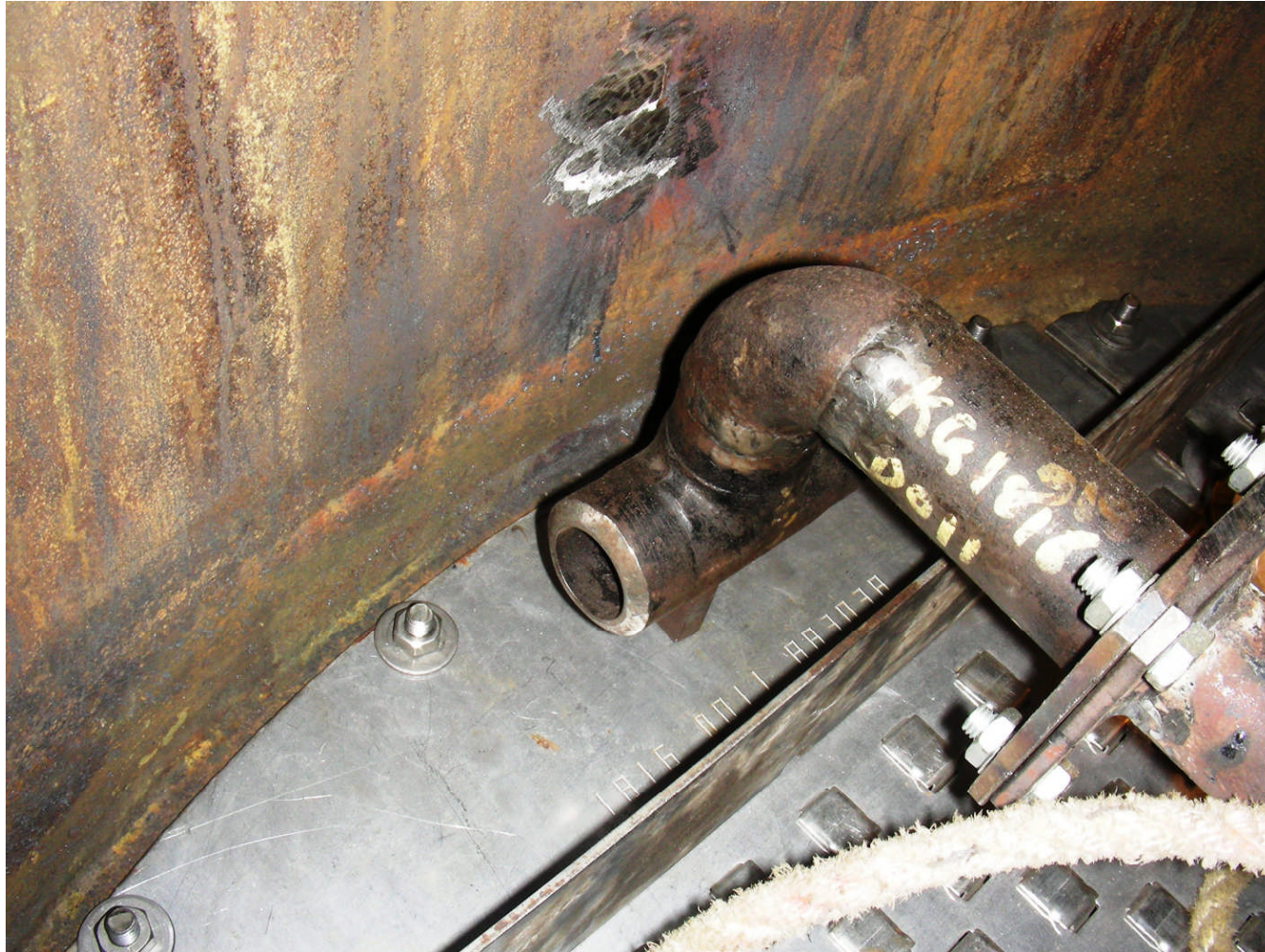
Reflux piping installed correctly
