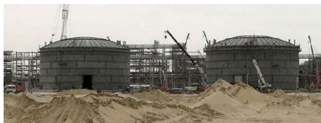
Figure 5 – Sadara 35m Wastewater Tank Construction (3)
