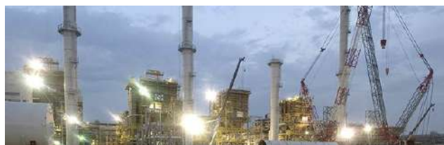
Figure 2 – Sadara Steam Boilers Under Construction (3)
